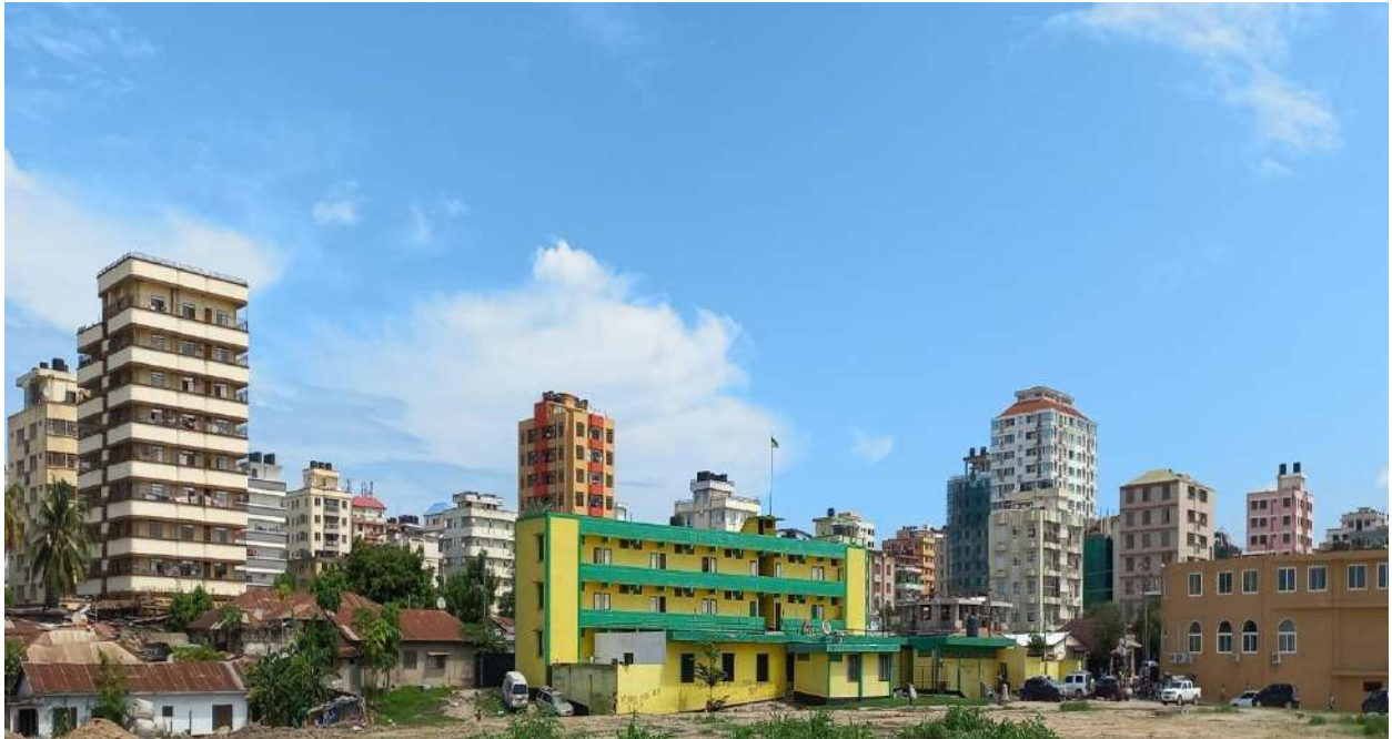
Figure 6-2: Some avoided structures in Kariakoo
