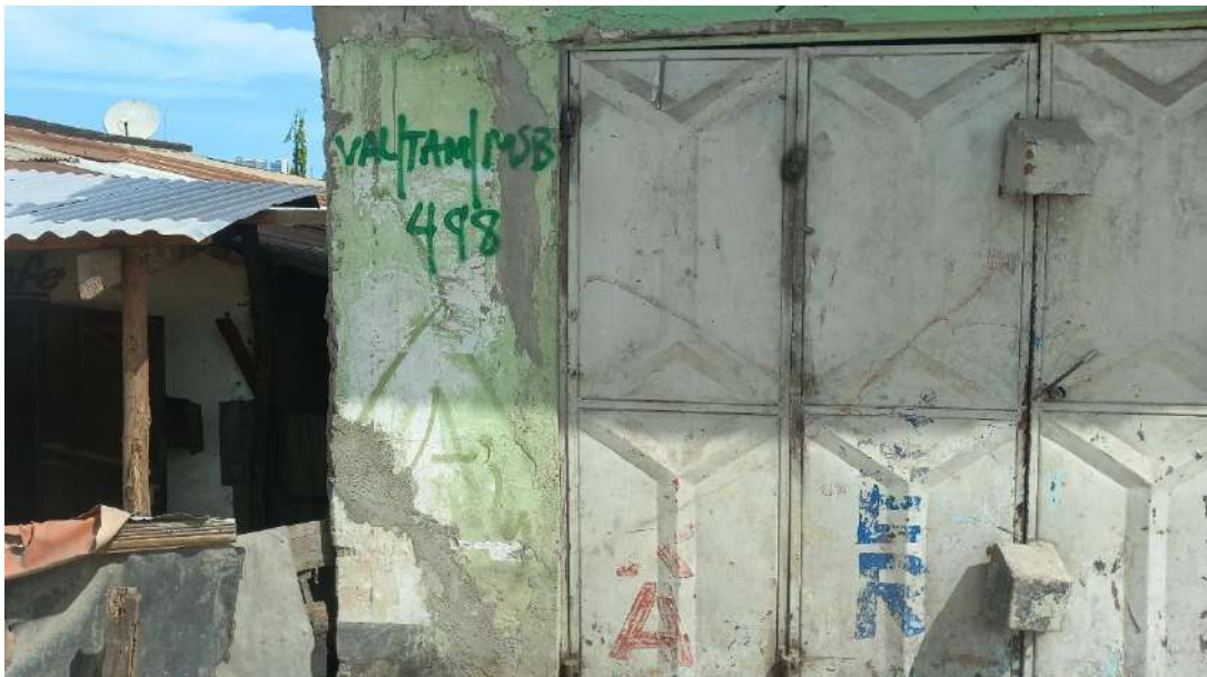
Figure 7-1: Example of marked structure
