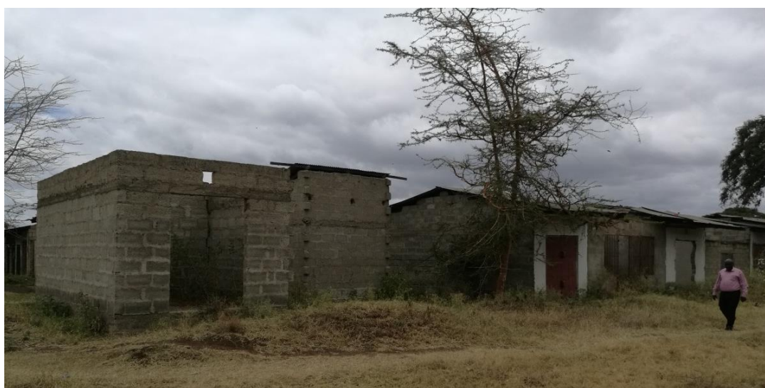
Figure 4: Unfinished Structures on the Plot
