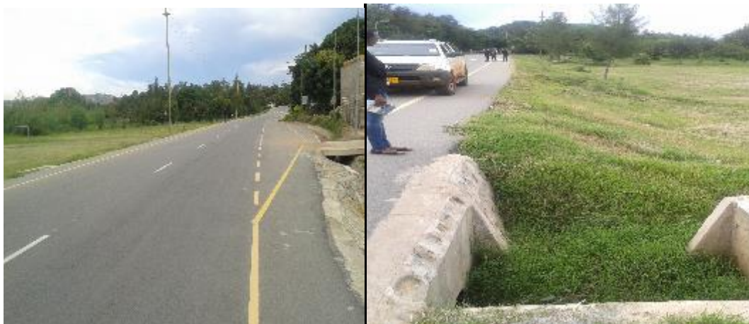
Figure 4.3: Existing conditions along the Butimba road
