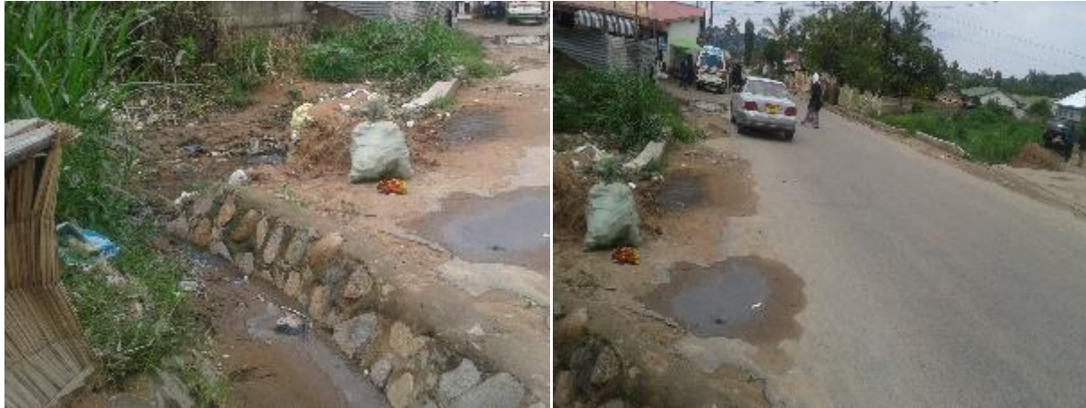
Figure 4.5: Existing Condition of River Msuka bank
