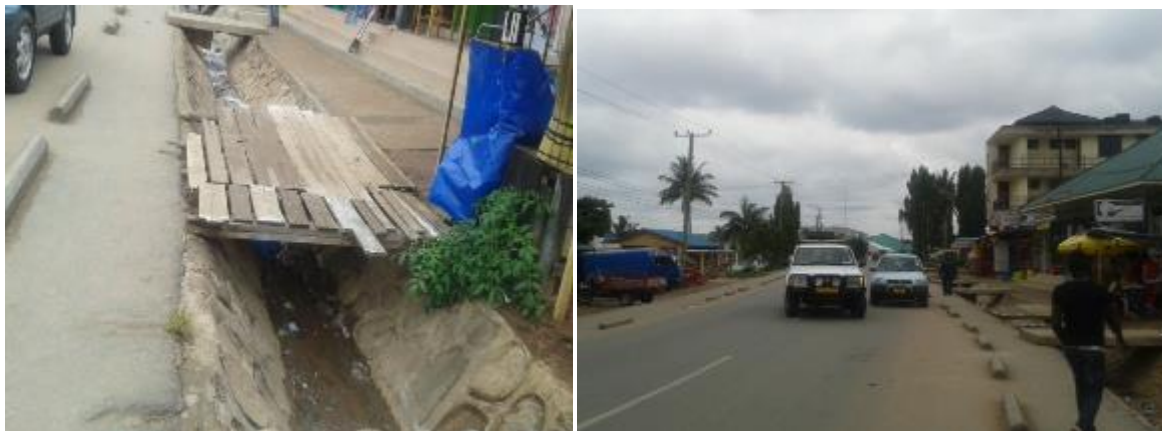
Figure 4.1: Existing situation of Pasiansi-Buzuruga road
