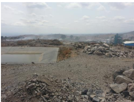
Figure 6: Smoke from burning waste, crashed rocks and leachate pond downstream of constructed cell at landfill site.
