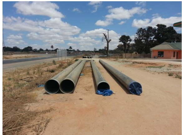
Figure 6: The laying of new water pipes in DMC
