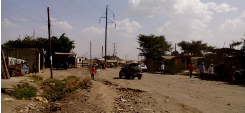
Figure 4.1: High tension power line traversing the road
