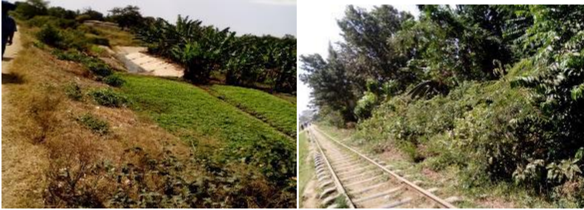
Figure 4.4: Conditions along the proposed Bondeni drain route
