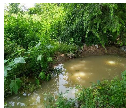
Lack of drainage and poor slope leading to water clogging
