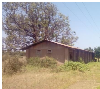
Unoccupied building on the Project site
