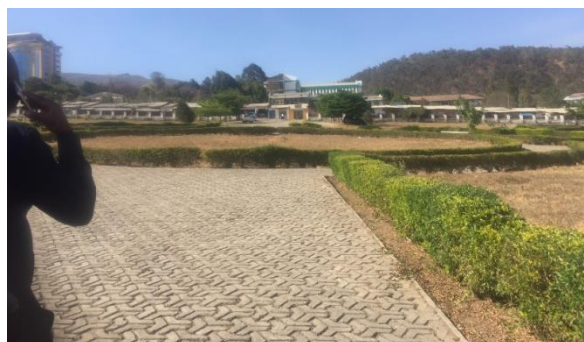
Figure 10: Existing structures at Mbeya City Park
